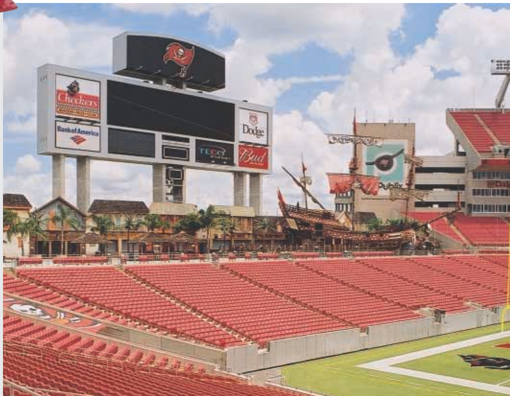
Raymond James Stadium, Tampa, FL – home of the Super Bowl XXXVII champion Tampa Bay Buccaneers. Construction Managers: Hunt Construction
