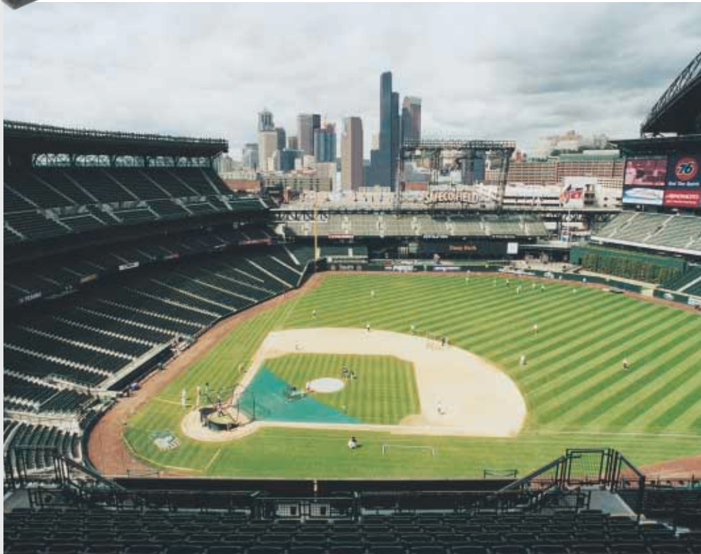
Safeco Field, Seattle, WA Construction Managers: Hunt Construction Architect: HNTB
